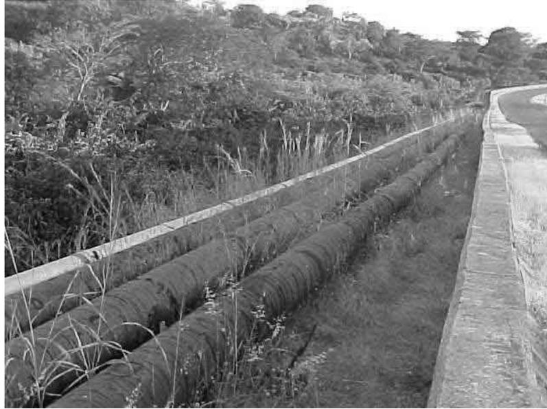
**Figure 1.1:** Typical oil steel pipeline coated with bitumen.
