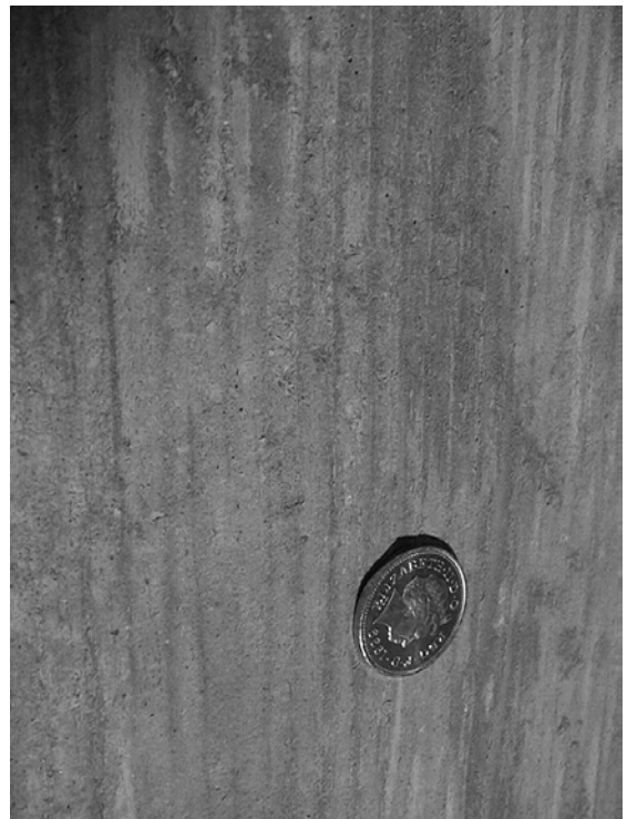
Figure 6.7b. Zoom in of timber shuttered surface.
