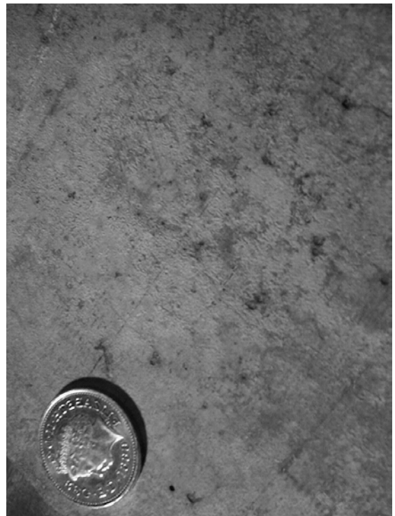
Figure 6.5b. Zoom in of flat surface concrete block.
