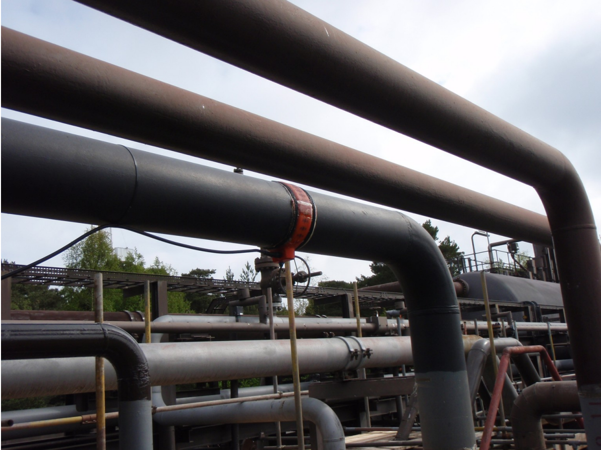
Figure 4.1: Example of a Guided Ultrasonics Ltd. gPIMS® sensor [20] installed on a pipeline.
