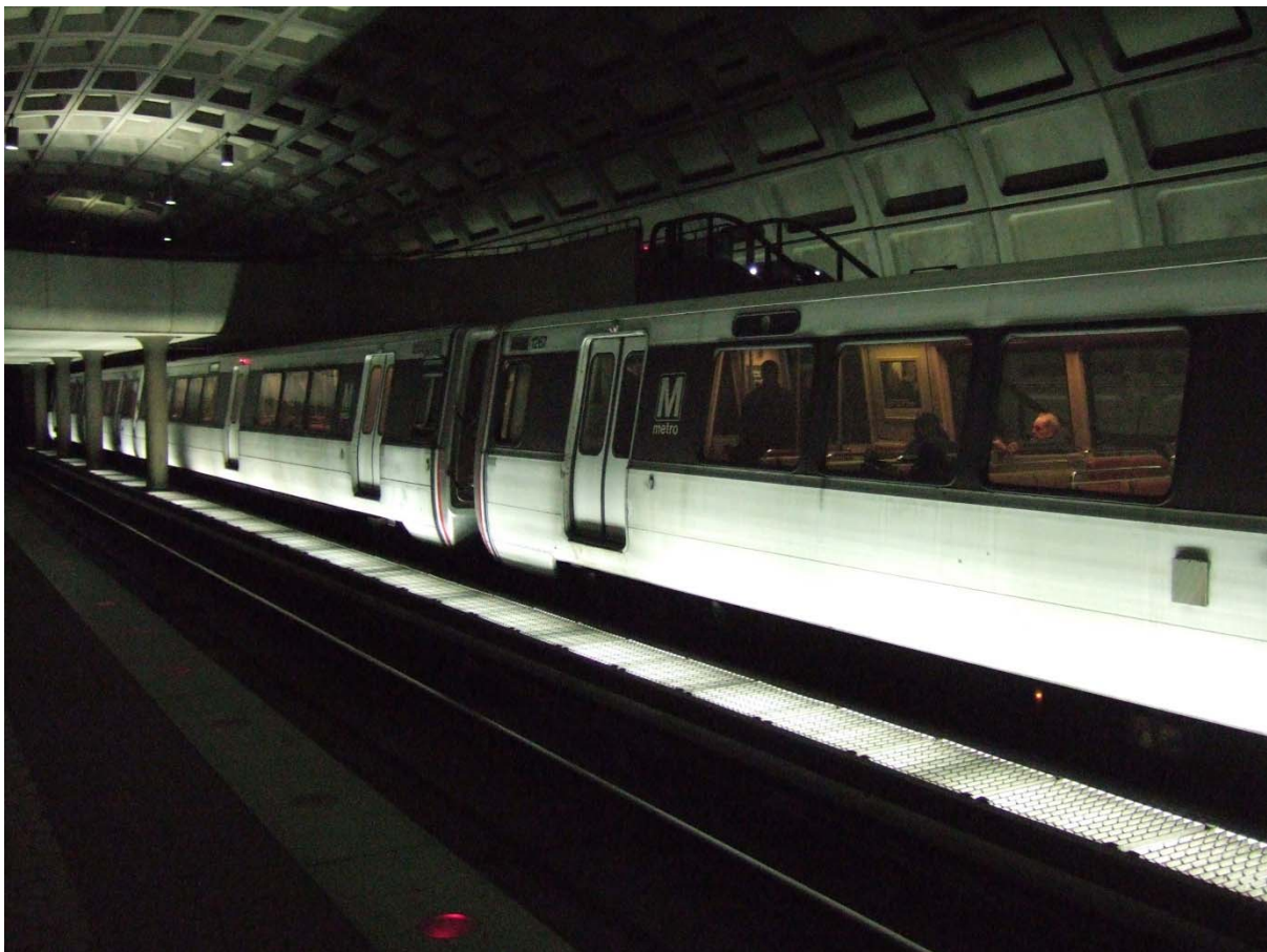
A WMATA station with lighting levels and round ceiling panels, making maintainability difficult
