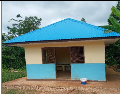
Photo 8: New permanent kitchen at Mtuhaliwa Primary School
