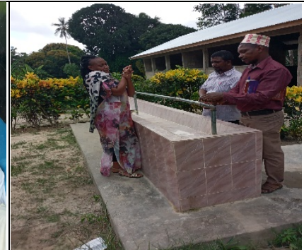
Photo 3: New constructed group hand washing at Maziwani School in Pemba.
