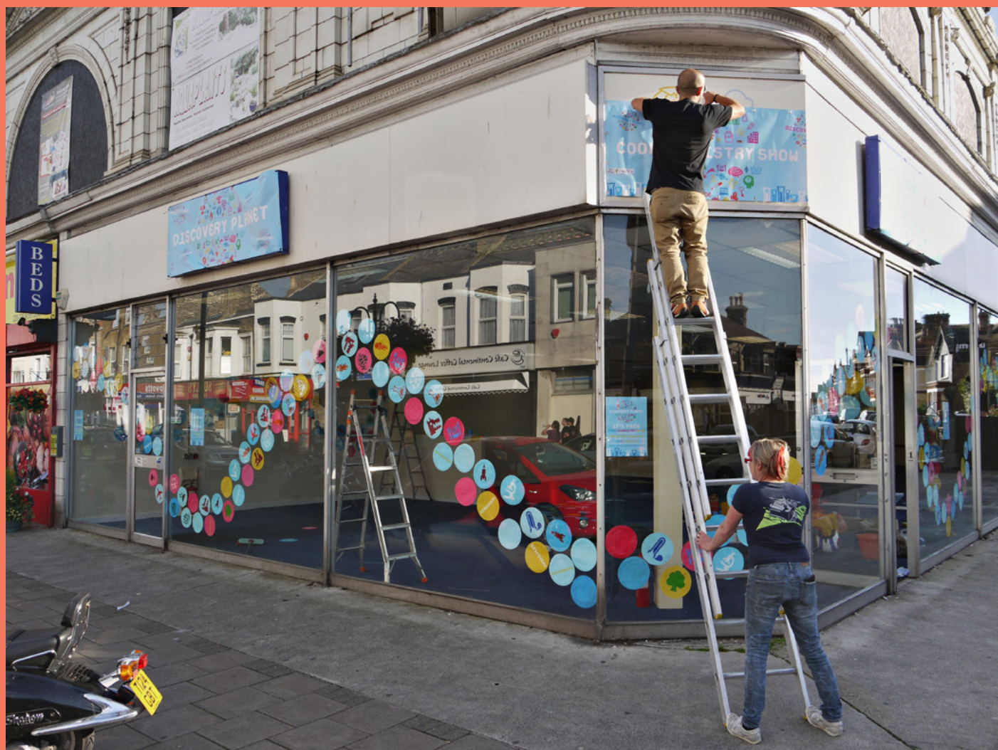
Transforming a former bed shop in Margate into Cool Chemistry
