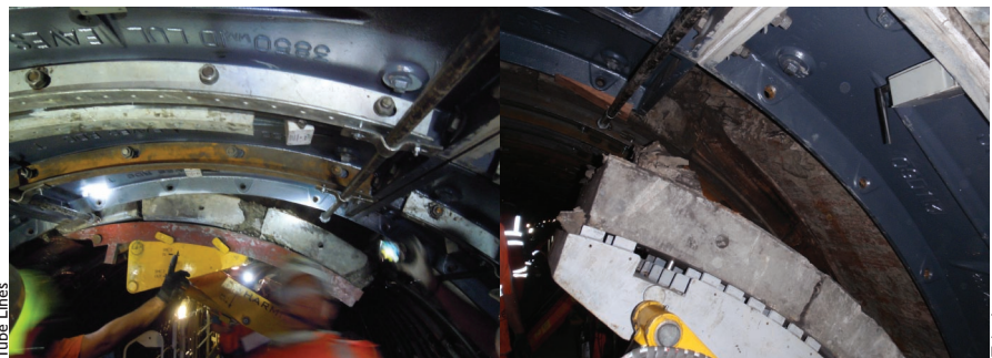
Tunnel lining replacement in action
