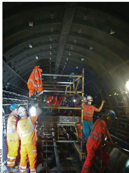
Sensors in place, ready to grout
