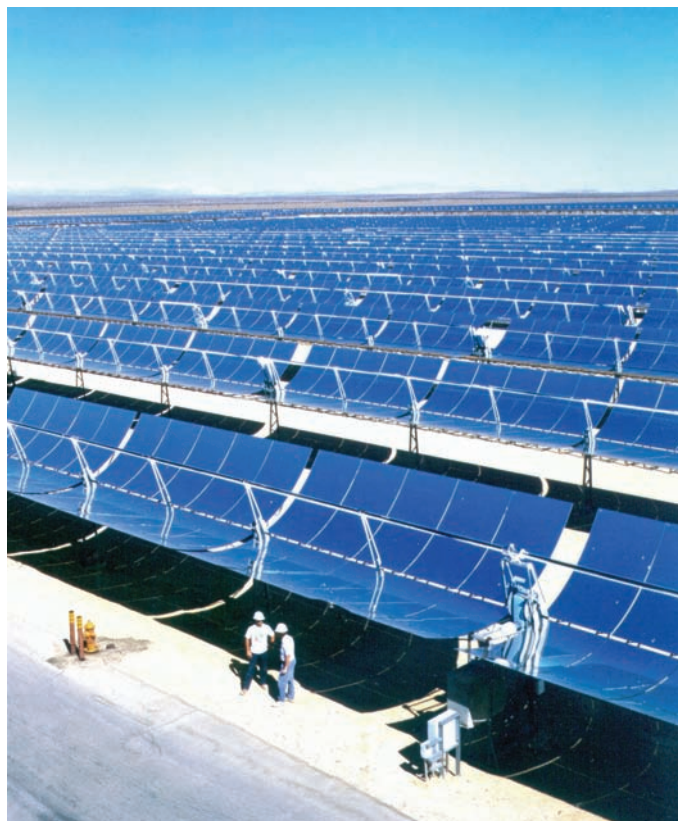
150 MW parabolic trough mirrors at Kramer Junction, California.
