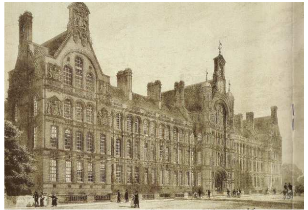
The (now demolished) City and Guilds building, Exhibition Road.
