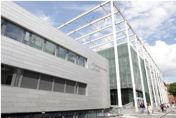
The Exhibition Road entrance to the College, including part of the modern City and Guilds building and Business School entrance.
