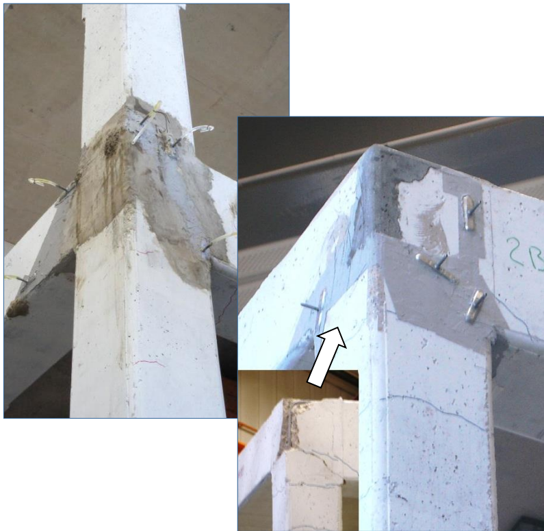
Crack injection & replacement of damaged concrete
