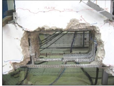
Removal of damaged concrete
