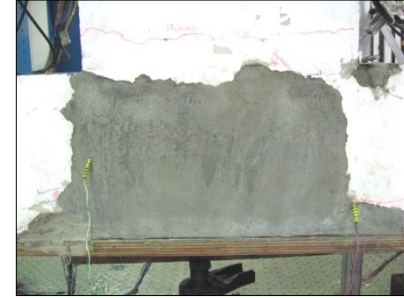
Re-casting using high-strength concrete
