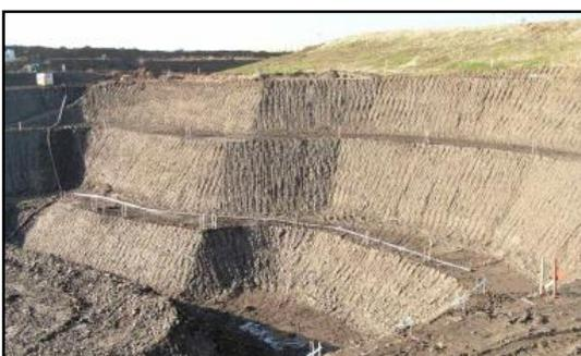
Figure 9. Heathrow Terminal 5 temporary excavations designed using ICFEP (Kovacevic et al., 2007)
