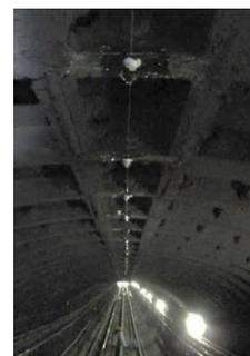
Figure 13. Use of optical fibres for monitoring existing Central Line tunnels during Crossrail tunnel construction beneath them
