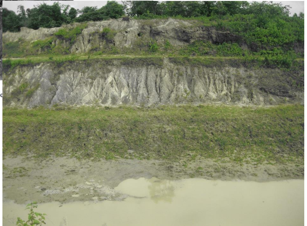
Sinthe dam: Outlet irrigation canal
