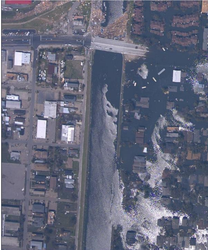
Breach in 17th Street Canal levee in New Orleans, Louisiana, on August 31, 2005
