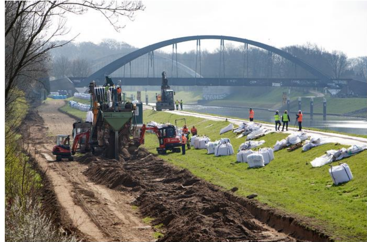
Strengthening of Twente Canal (Twentekanaal)
