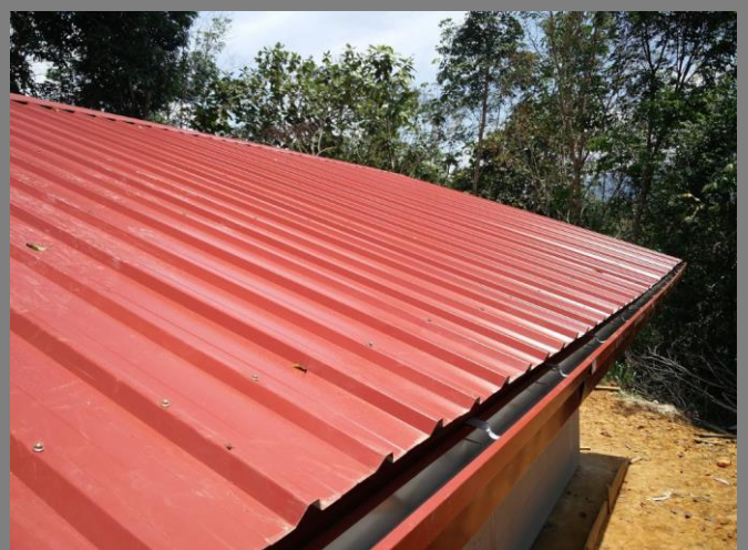
Figure 30: Gutter and fascia.
