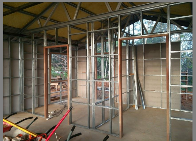
Figure 33: Internal wall studs
