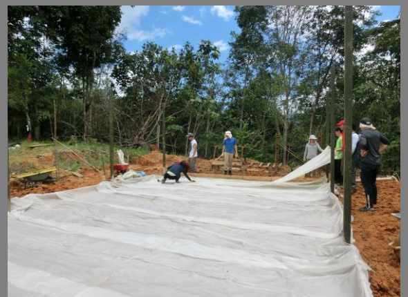
Figure 27: Concrete slab water proofing.
