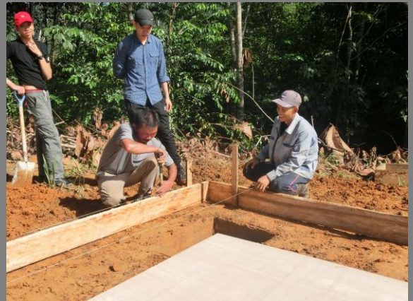
Figure 20 Setting out.
