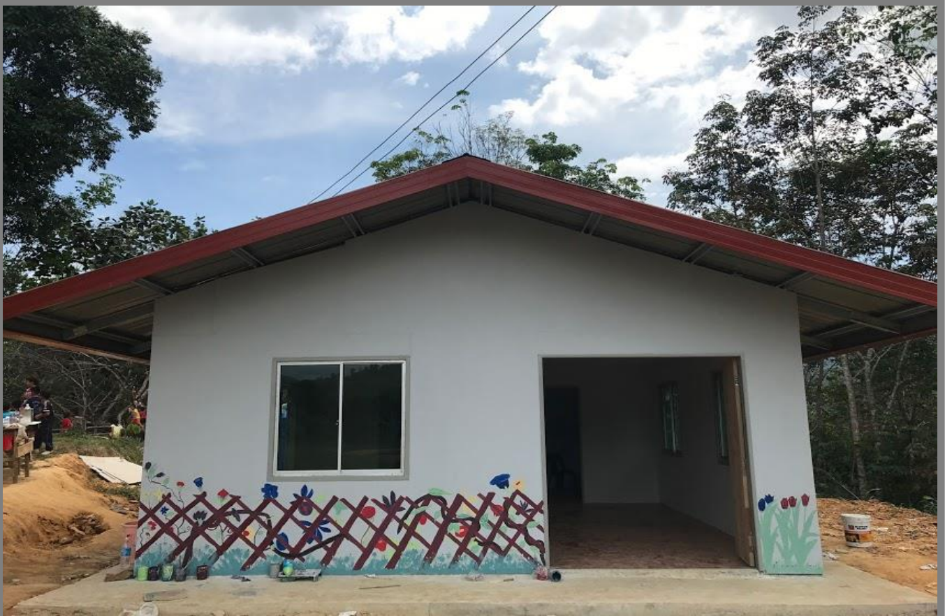
Figure 19: Façade of the kindergarten.
