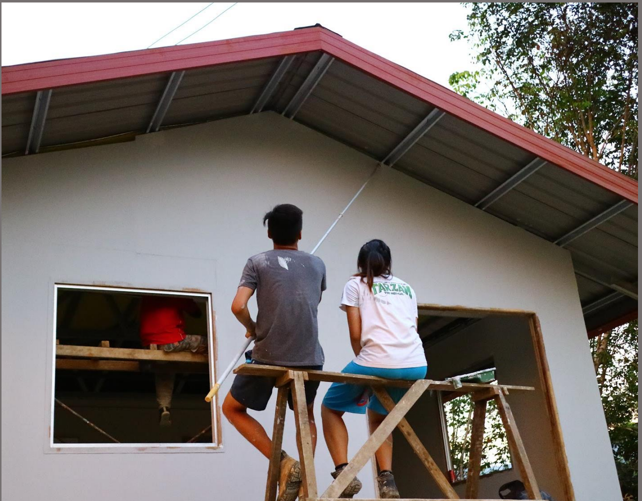
Figure 14: Jeffrey and Shi Jinn painting the prefabricated cement wall panels.
