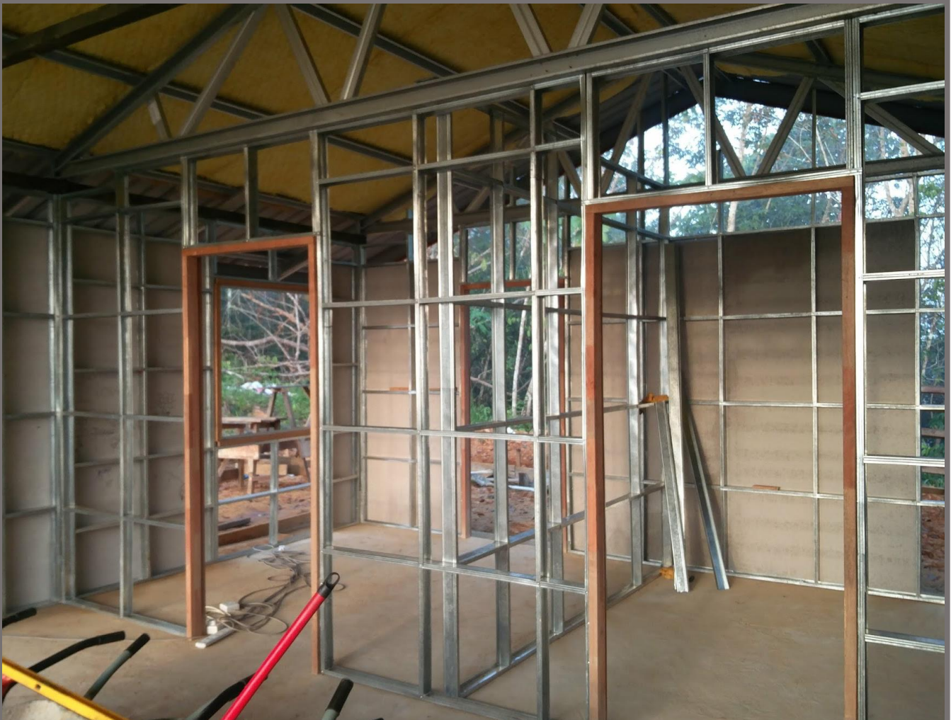
Figure 13: Internal wall frames of the kindergarten.
