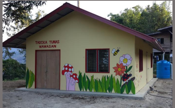
Figure 6: Kindergarten completed in Ranau, Sabah.
