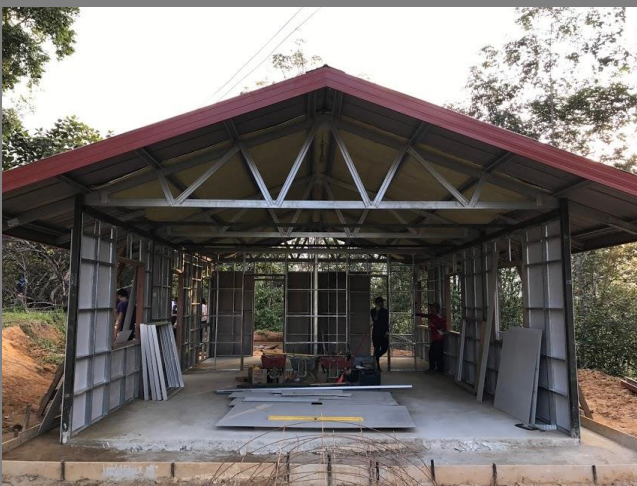
Figure 32: Wall studs overview.
