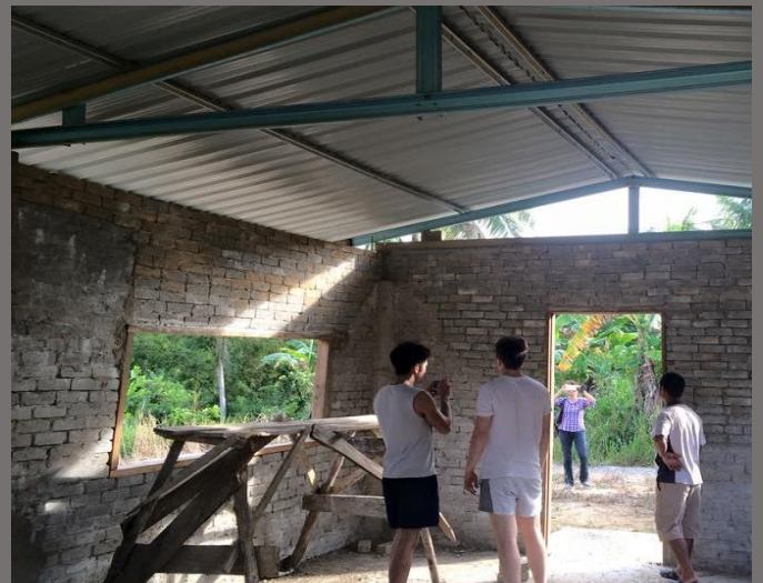
Figure 4: Edrea and Jack surveying a construction site.
