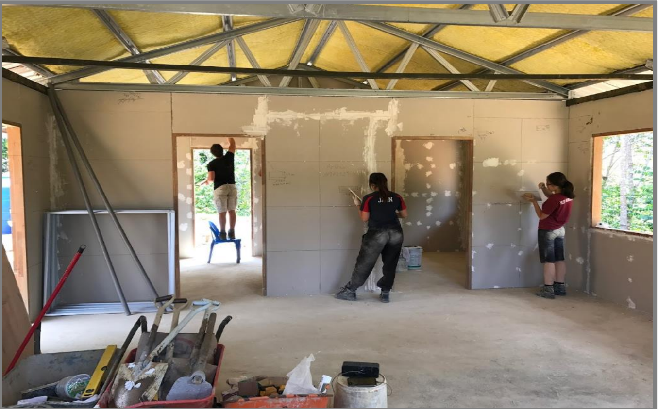
Figure 37: Plastering the wall panels.
