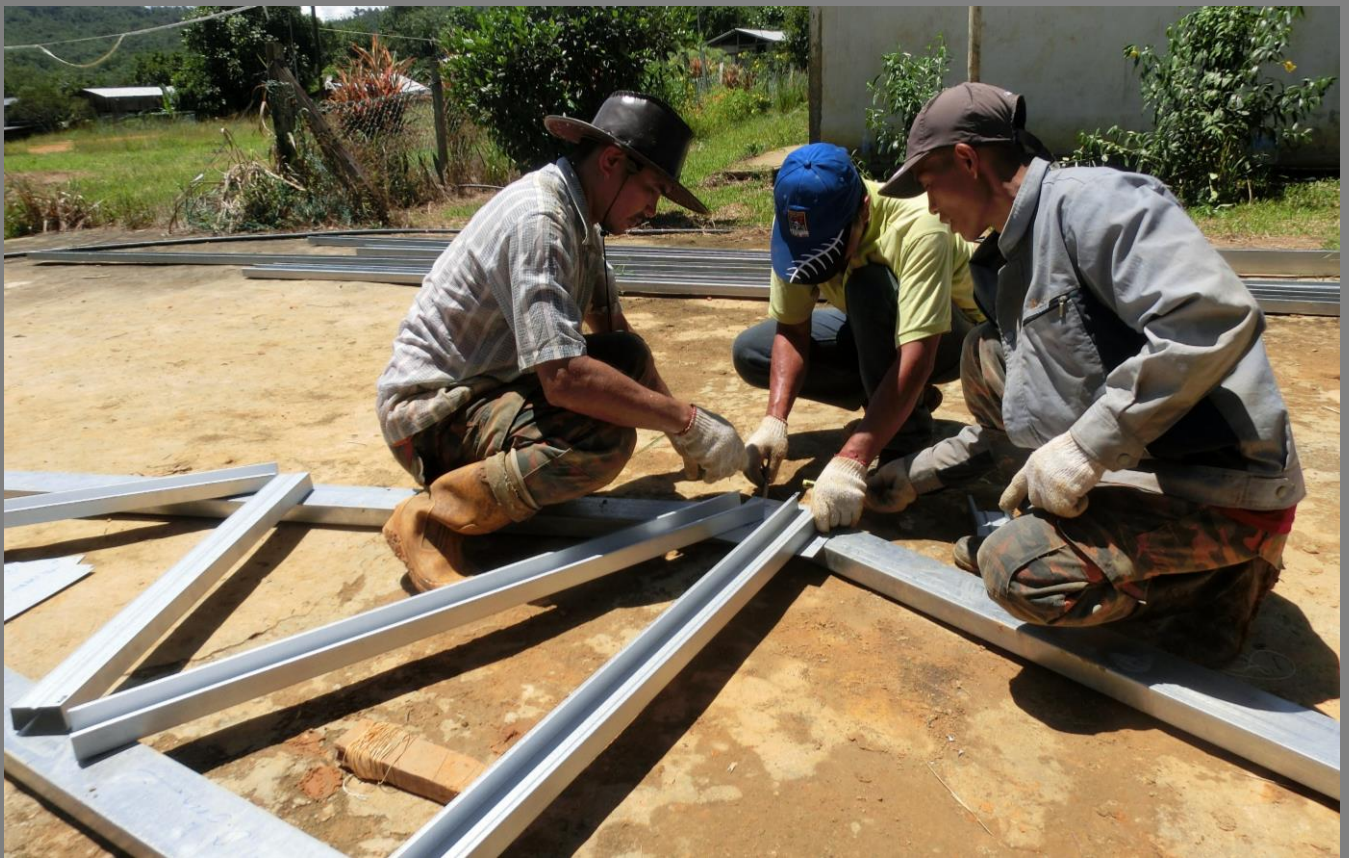
Figure 25: Truss assembly.
