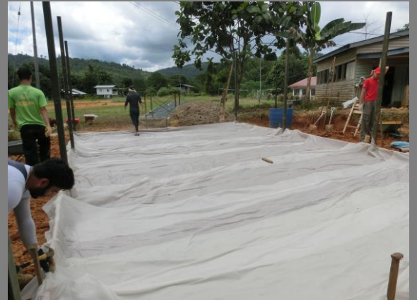
Figure 26: Polyethylene sheets positioning.
