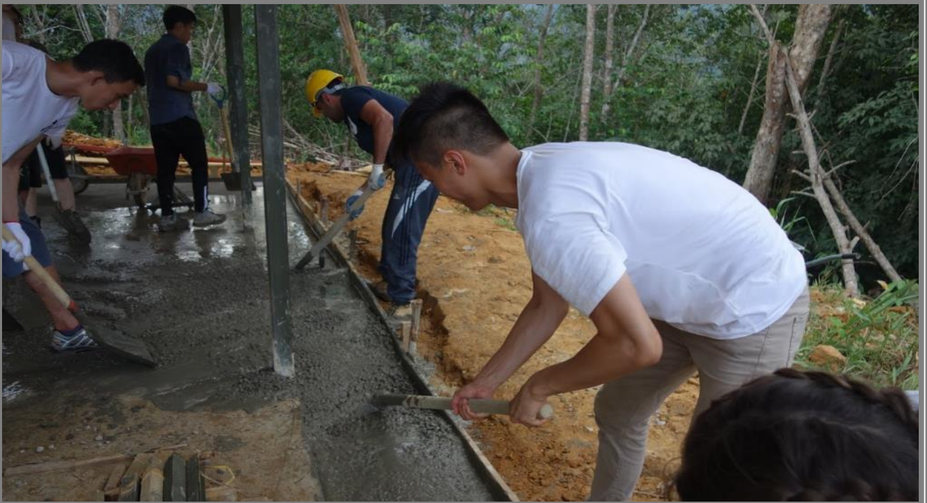
Figure 28: Casting of the outerslab.
