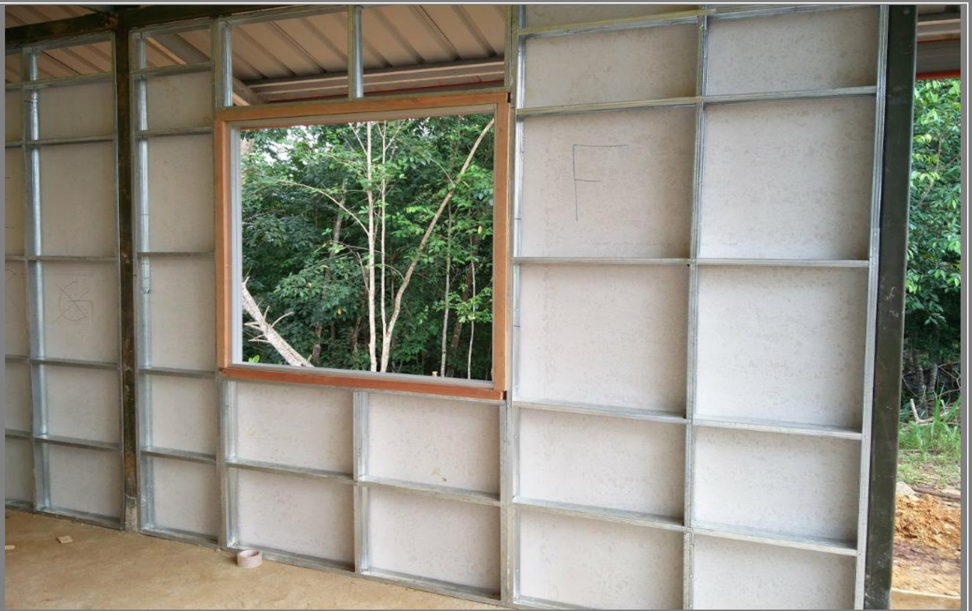
Figure 31: Wall panels attached onto the wall studs.
