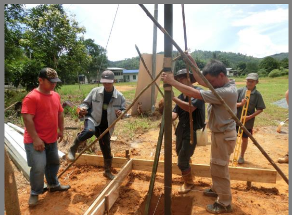
Figure 21: Column propping
