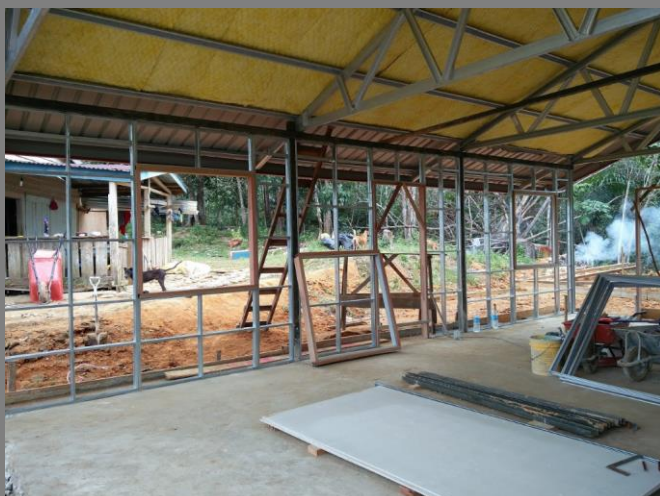
Figure 29: Wall studs.
