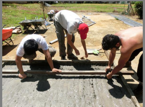
Figure 23: Spacer making
