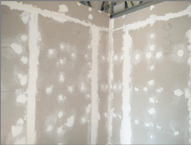
Figure 37: Plastering the wall panels.
