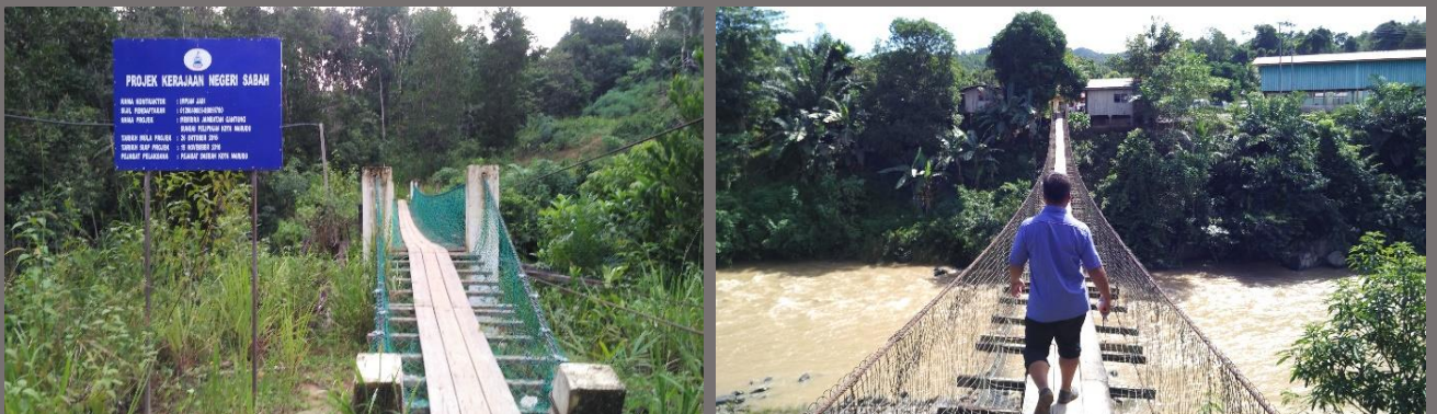
Figure 8: Hanging bridges that span Sungai Palipikan (L) and Sungai Kanarom (R).
