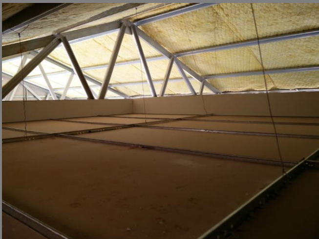
Figure 38: Ceilings suspended from the battens
