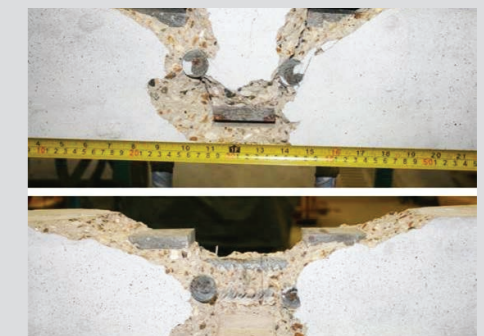
Failure of 3 bar headed bar tension splice.
