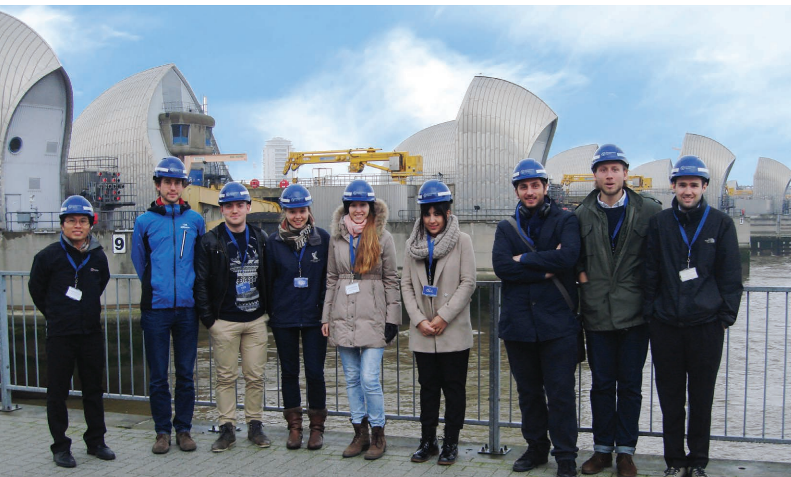
CDT students from cohort 1 visiting the Thames Flood Barrier as part of their Grand Challenge Project. The aim is that Grand Challenge Projects mimic the way leading companies in the Sustainable Civil Engineering sector address major problems, providing additional skills and training to students
