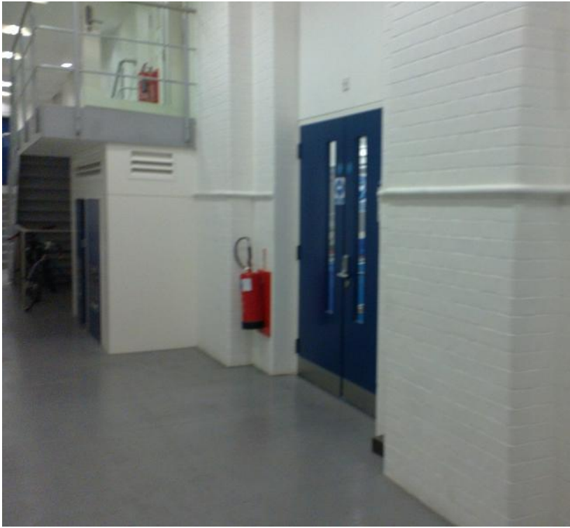
Workshop is then second blue doors on the right before the stairs
