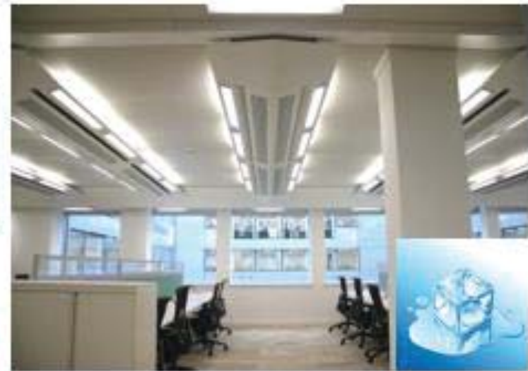
Chilled Beams
