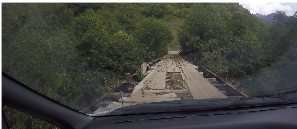
Figure 39. The questionable bridge to the put-in
