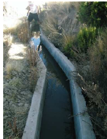
Concreted irrigation channel
