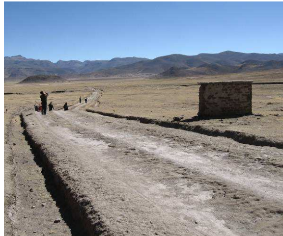
The dirt road constructed by the community
