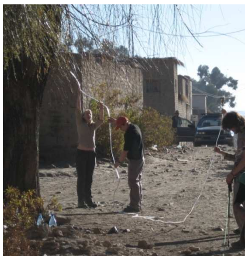
Getting bubbles out of the hosepipe before levelling
