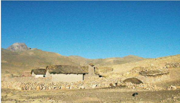
Adobe houses in Cortaviento
