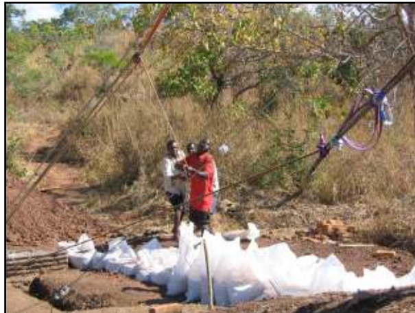
Fig. 3 - Three workers haul the walkway cable (right) over the west tower.
