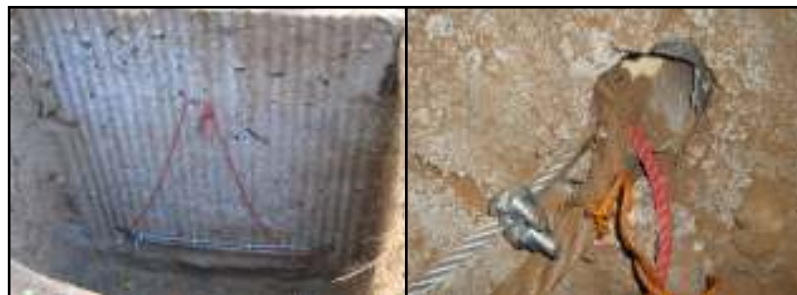
Fig. 2 – Access pit behind the eastern anchor block (L) and close up of the cables running through the plastic pipe set in the anchor (R). The red rope was left running through the plastic pipe to prevent it becoming blocked. The orange cord and grips mark the middle section of the walkway and handrail cables respectively.
