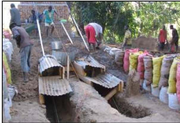
Fig. 7 – Building the embankment. Earth brought from stockpile (right) by wheelbarrow and sacks was spread out with hoes and compacted by hitting with shovel or jumping up and down on it (man to the right of wheelbarrow).
