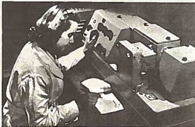
An example of Glaxo Analytical Control in action. Above, an analyst extracts vitamin A from a Vitablend animal feed supplement to check that the amount present corresponds to the declared formula. It is measured precisely in the ultra violet spectrophotometer seen below.
