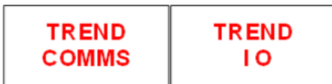
Figure 13 – Labels for BMS field and network cables
