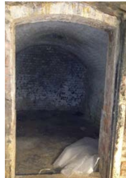
LEFT. TOP: THE REFURBISHED VAULTS, INSET KIRSTY SCALLAN, BOTTOM: THE PLANT ROOM. THIS PAGE: ABOVE: UNDER CONSTRUCTION. BELOW: ONE OF THE ORIGINAL COAL HOLES, RIGHT: THE CORRIDOR SHOWING THE MEMBRANE SYSTEM WITH THE BLUE FIXING POINTS, AND UNDERFLOOR DRAINAGE.
