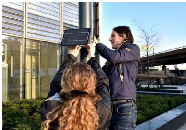
Image: Installation of Breathe London nodes is straightforward: they can be attached to a pole, post or wall using brackets and fixings and must be south-facing.
